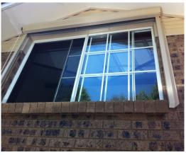
The Warrior Fire Shutter FZ range was designed and engineered as a neat solution to meet requirements of AS3959.4. The Warrior range is approved for at least 30 minutes fire protection (-/30/-). It is also made in Australia by a 100% owned and operated Australian company.
